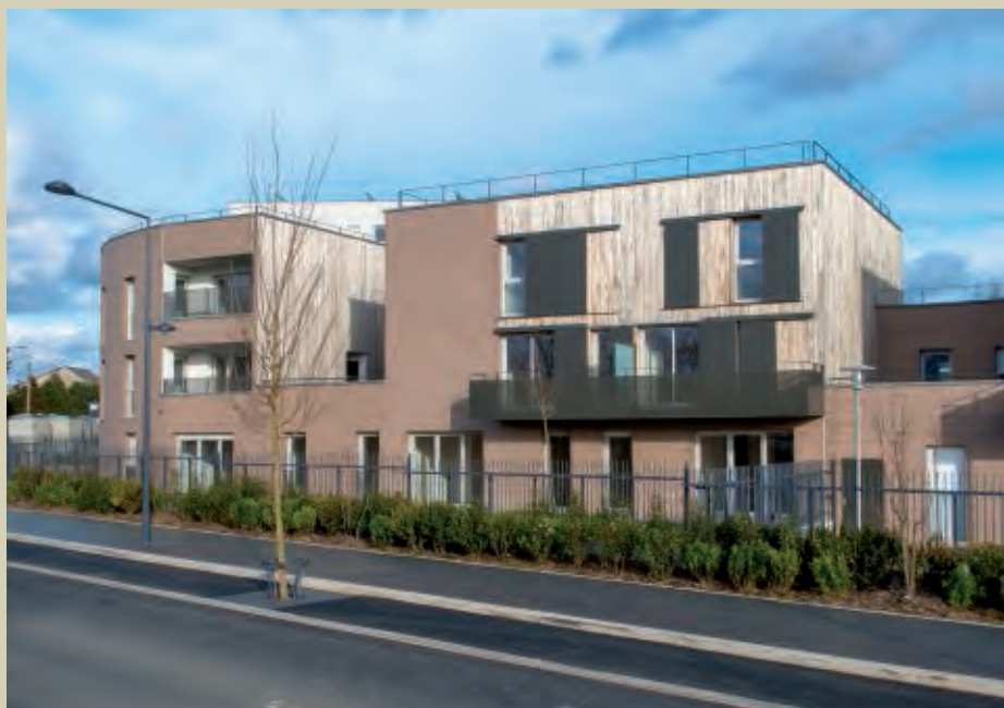
Stains, PRU Le Clos Saint-Lazare, construction neuve George Sand.
